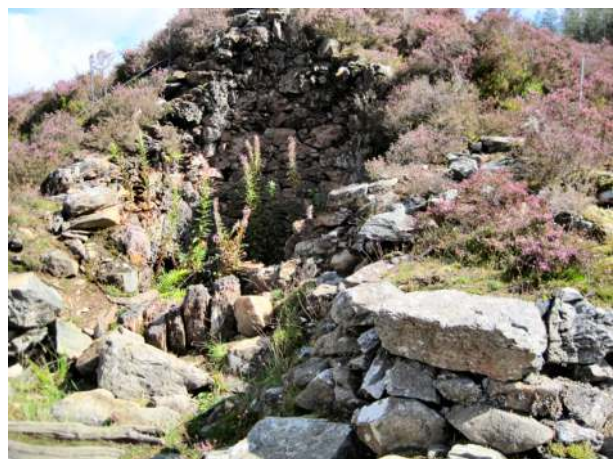
The remains of a kiln used to ash the copper bearing peat at Turf Copper Mine. G. Morse photograph, September 2010.
